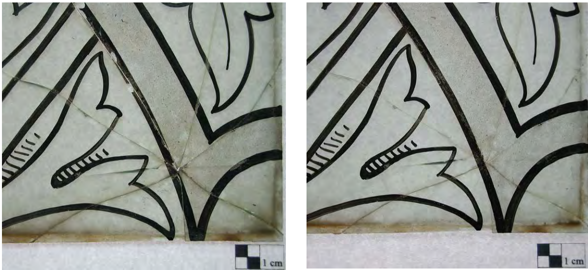
Figure 9: Detail of one grisaille fissure area before (left) and after restoration (right).
