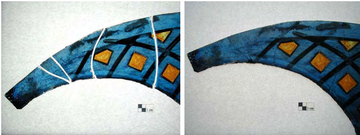
Figure 11: Round window from the Bethmann Hollweg grave chapel in Hohen Finow/ Brandenburg from 1893, before (left) and after restoration (right), cracks were filled with clear Araldite while the parts flaked off were filled with the “adhesive-glass-powder mixture”.
